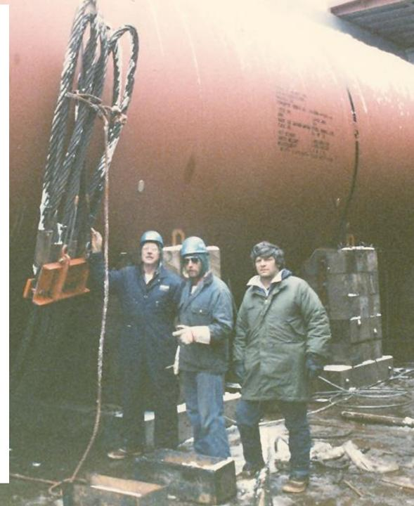
Using the special spreader bar to hook up the four slings Special hook up spreader bars
