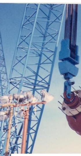
Flange lug with a temporary work platform built around it
